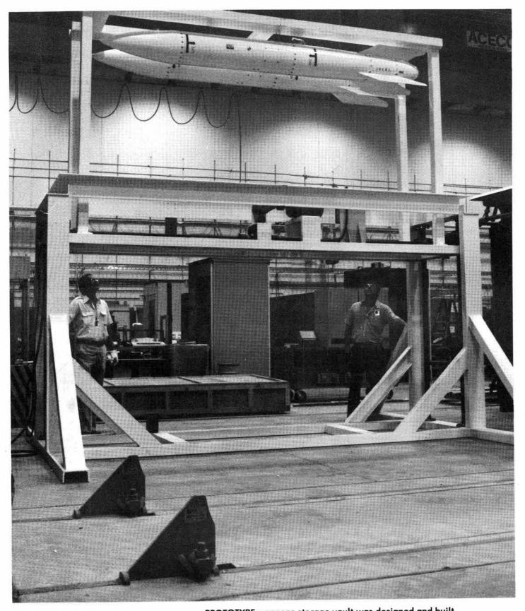
PROTOTYPE weapons storage vault was designed and built by Dept. 1720 and is being evaluated by the Air Force for use at its bases. Work falls under safeguards program.
